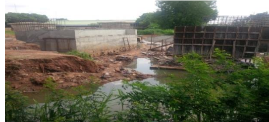
Plate 6. the on-going construction of bridge at coca-cola road.
