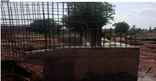
plate 5. the on-going construction of the bridge at coca-cola road.
