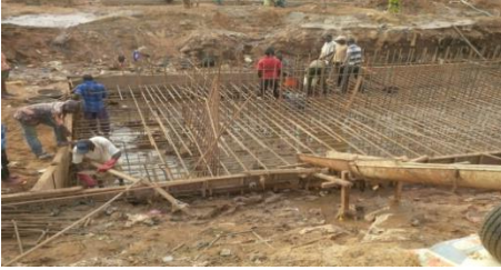
Plate 1. Arrangement of reinforcement bar
