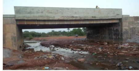
Plate 2. The new constructed bridge at Ajegunle-egbejila road.
